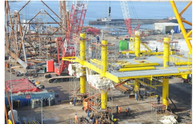
Works performed on Akcakoca Project
